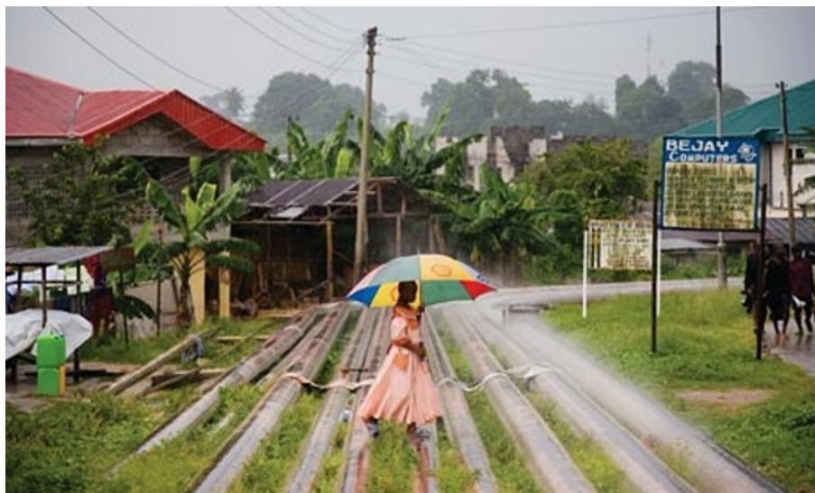
Oil Pipelines in Okrika, Nigeria (source: theguardian.com)
